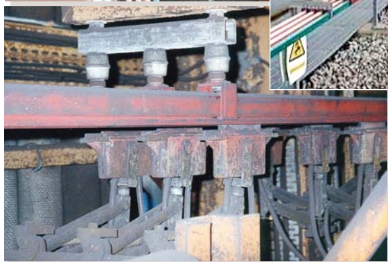
300 metres of 800A bar ↑ → with medium heat cover feeding two steelwork cranes. Dusty, corrosive and hot (+80°C) environment. Using insulated hanger clamps supplied pre-fitted to support brackets.
