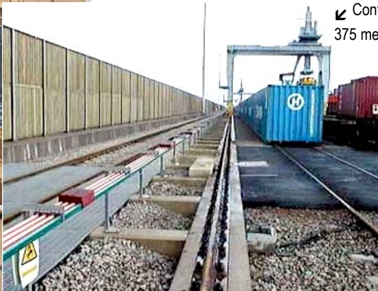
← 3 cranes operating outdoor on a 456 metres system, comprising 3 x 1250A Phase and 1 x 800A Earth conductor.
